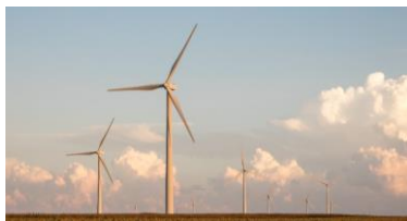
Invenergy's Grand Ridge Wind Energy Center located in LaSalle County, Illinois.
